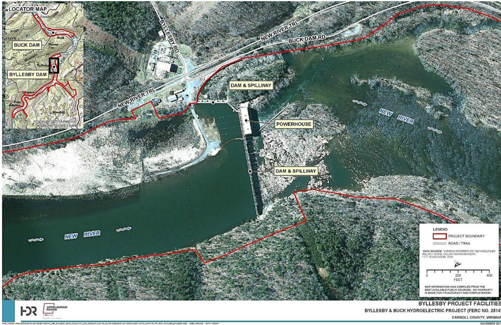
Figure 1-2. Byllesby Project Facilities
