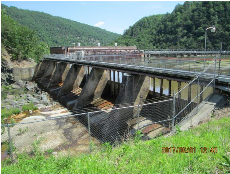
Photo 4.3-3 Byllesby emergency spillway dam
