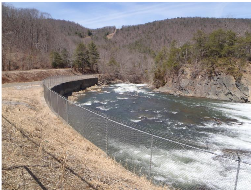
Photo 4.3-4 Flows through Byllesby emergency spillway channel during operation in March 2014
