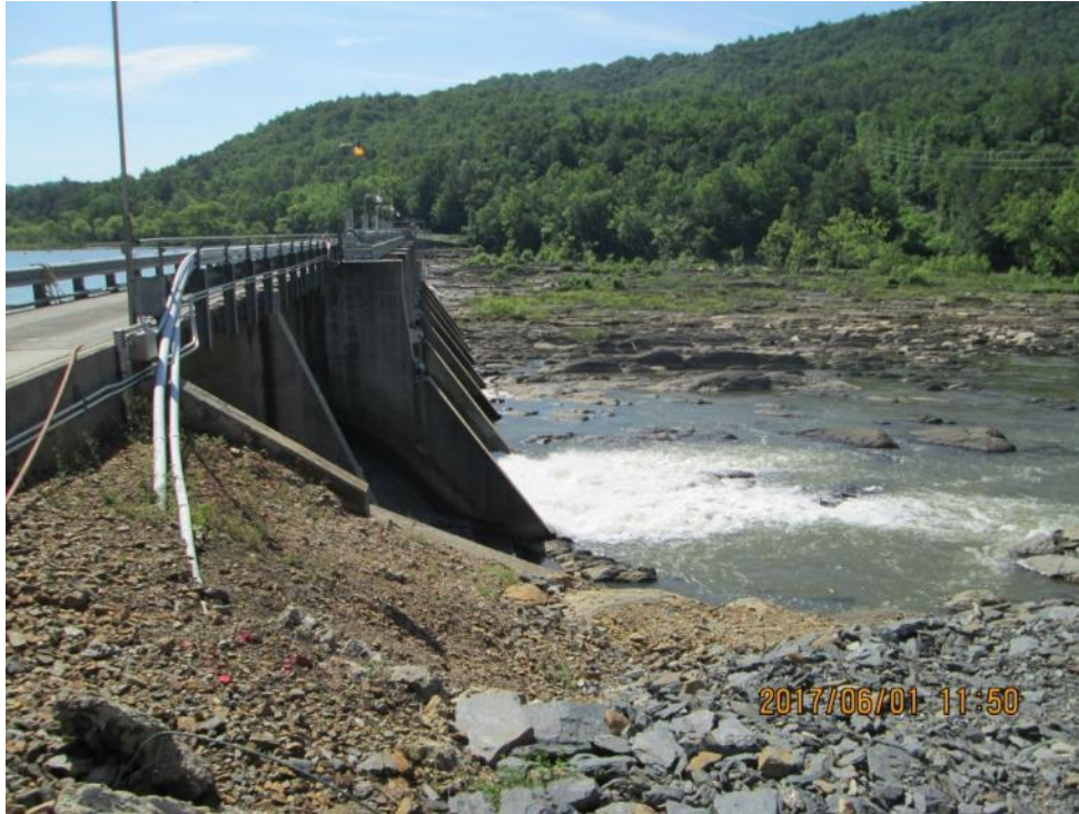
Photo 4.3-6 Buck spillway gates
