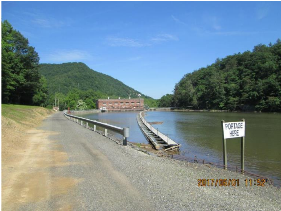
Photo 4.3-5 Buck powerhouse, log boom, and main dam, as viewed looking downstream from reservoir
