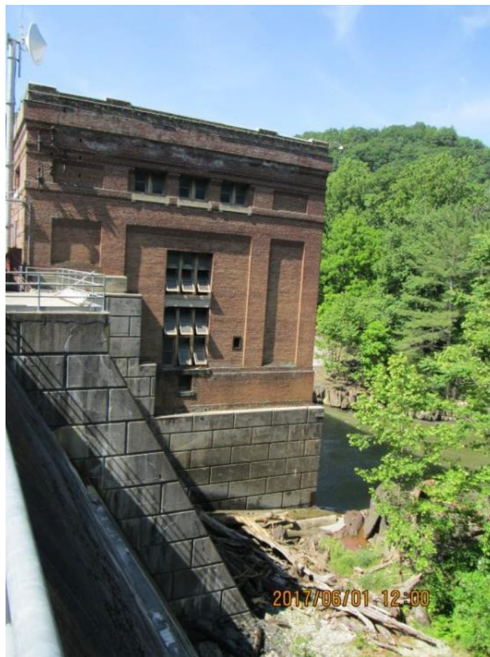
Photo 4.3-10 Buck powerhouse and tailrace
