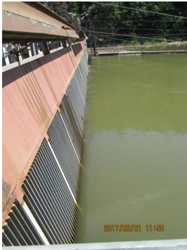
Photo 4.3-7 Buck intakes and trashracks
