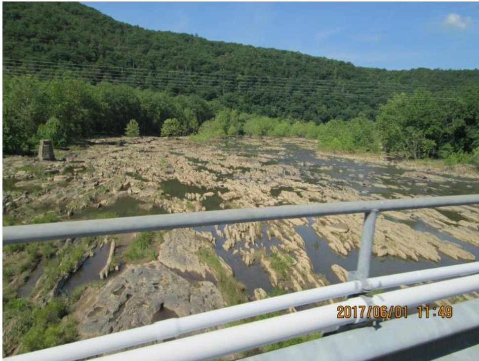
Photo 4.3-8 Buck bypass reach, as viewed looking downstream from the gated spillway
