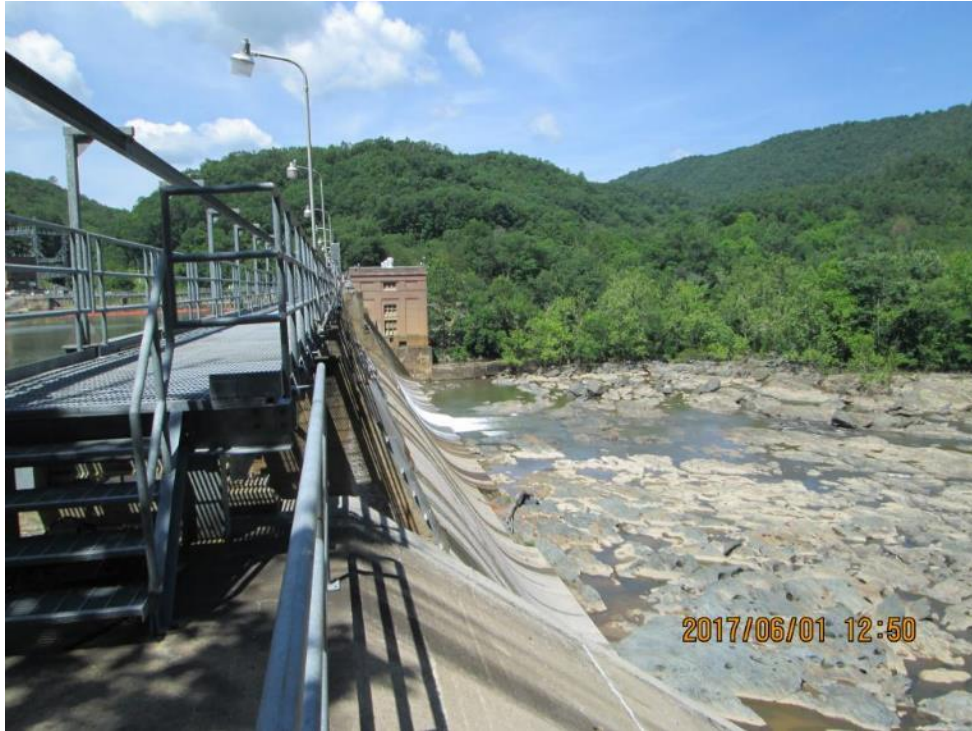
Photo 4.3-2 Gated section of Bylesby spillway
