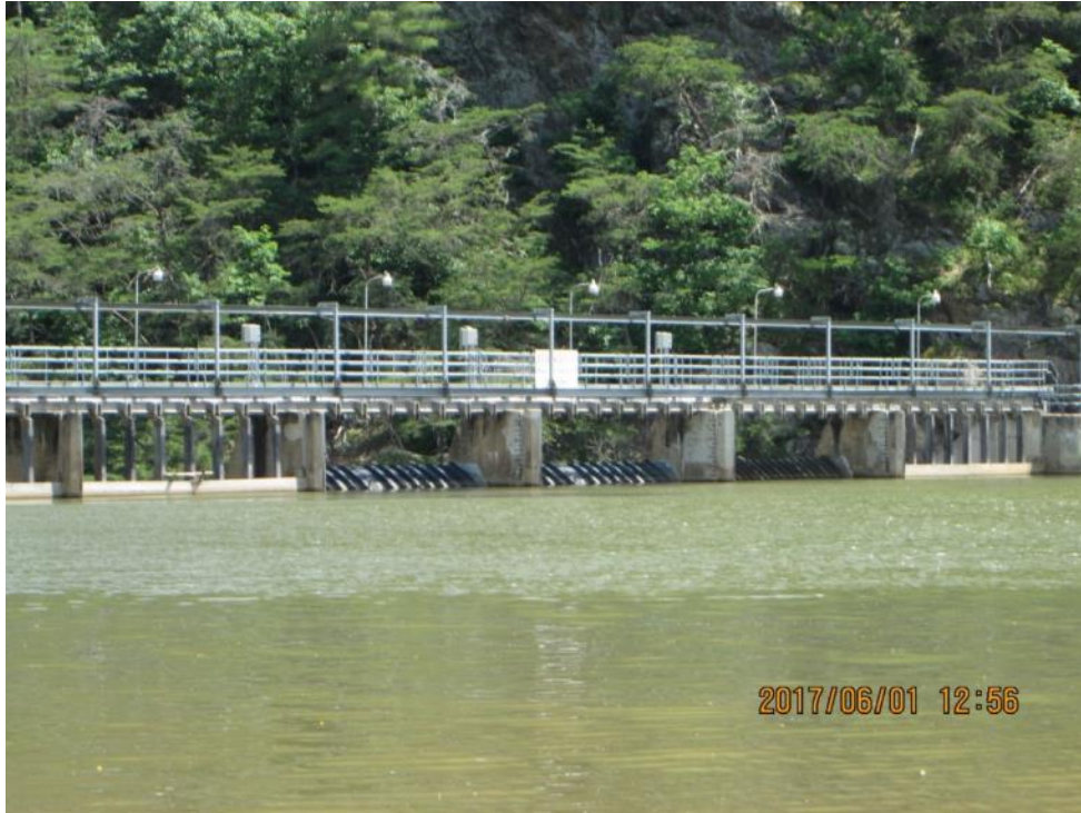
Photo 4.3-1 Obermeyer crest gates at Byllesby spillway
