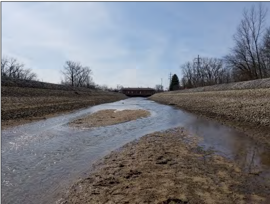
Figure 3. Representative photo of exposed bars and approximate final minimum water level achieved within the head race channel on April 2, 2019. Photo taken approximately 800 feet upstream of power house, facing downstream.
