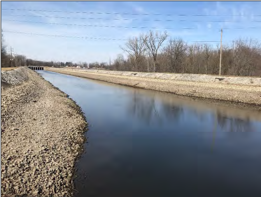
Figure 2. Water level in the head race channel on March 27, 2019. Note stone on channel banks and channel bank toe-of-slope just starting to become exposed. Photo taken at downstream end of head race at power house, facing upstream.
