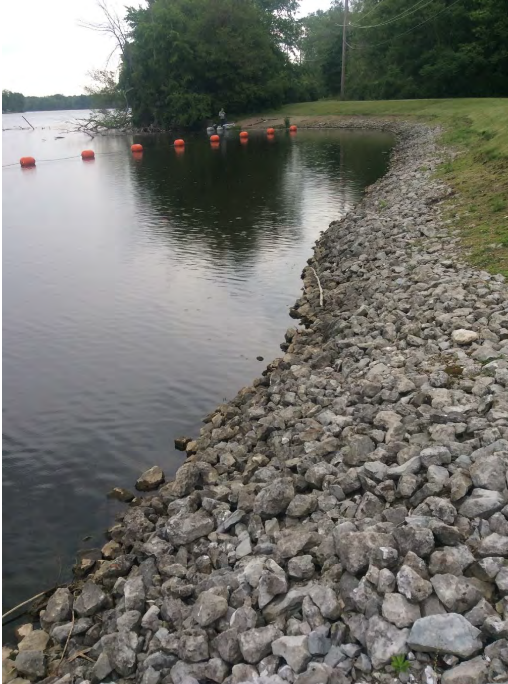
Figure 9. Site SJR45: Example of shoreline armoring.
