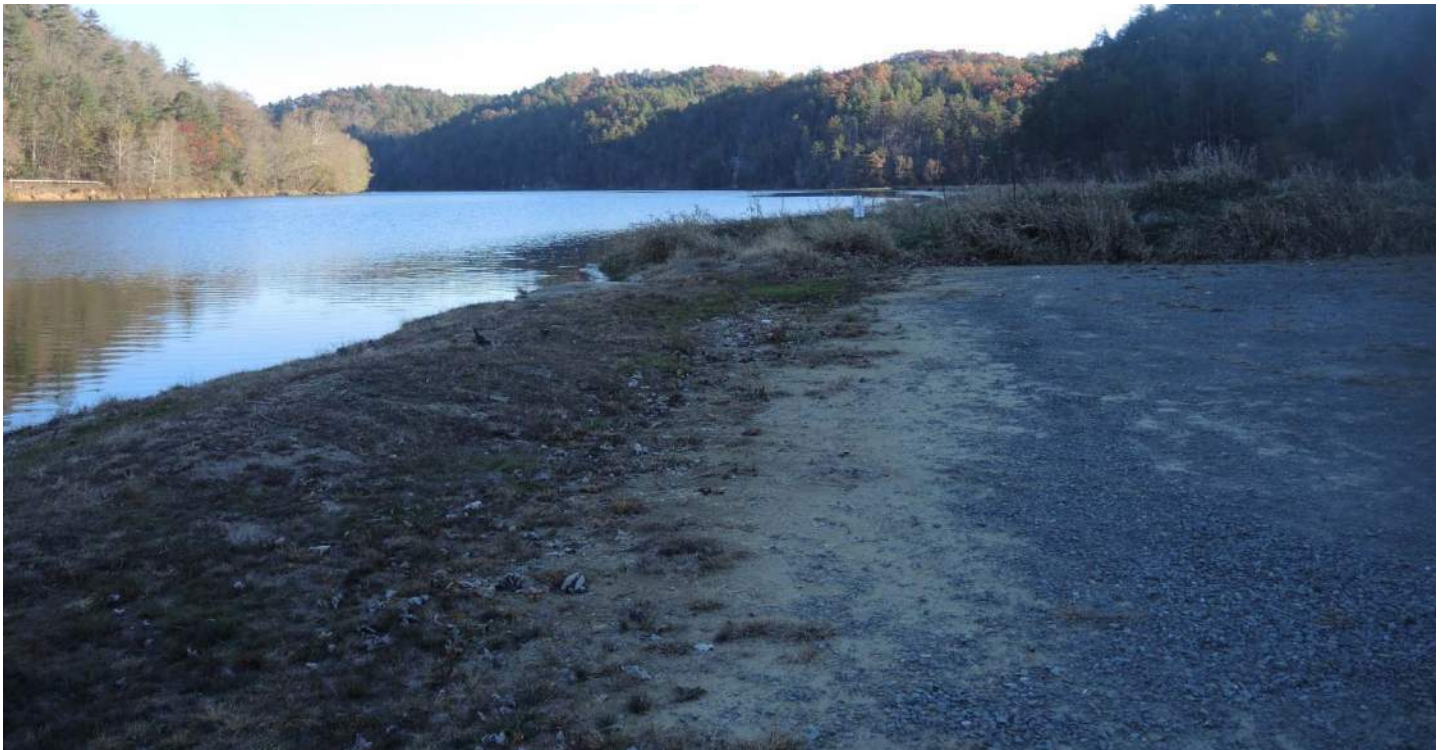
Photo 1-4: Soft dirt edge along parking lot
