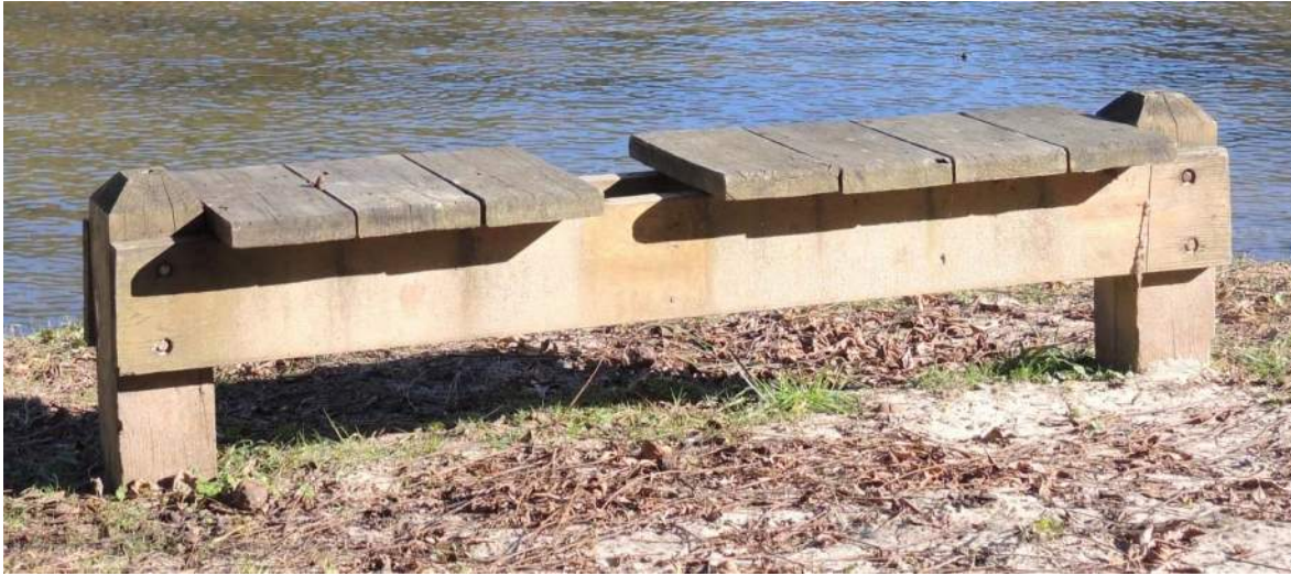
Photo 5-9: Bench with missing slat
