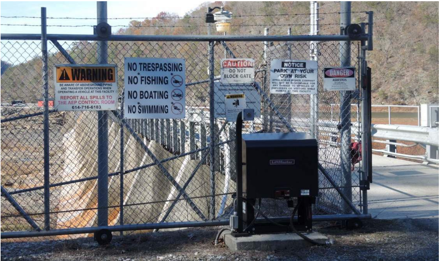
Photo 6-2: Dam gate with regulatory signs
