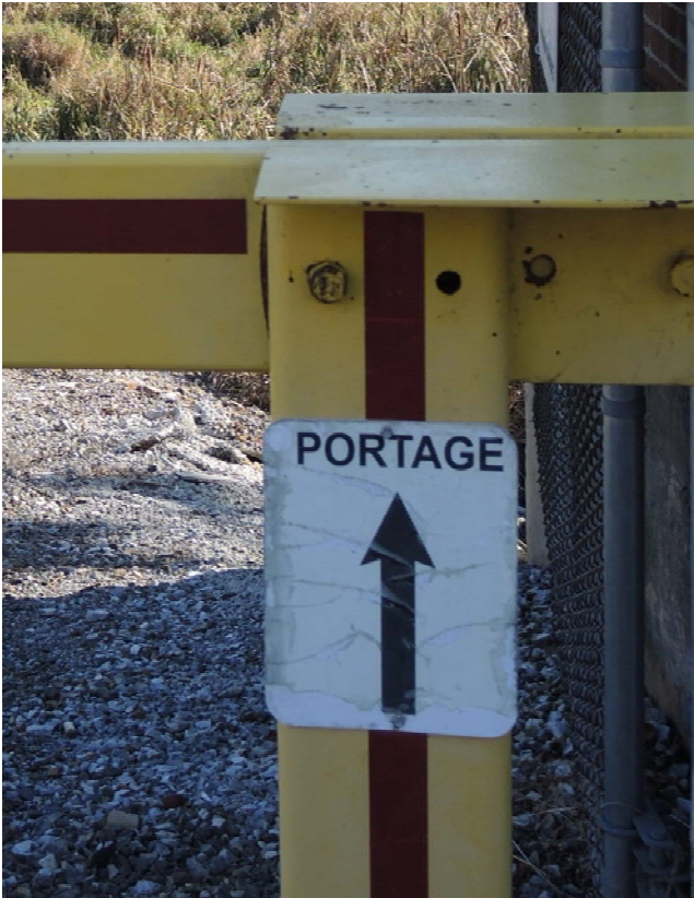
Photo 3-6: Portage sign on gate is very small and cracking/peeling
