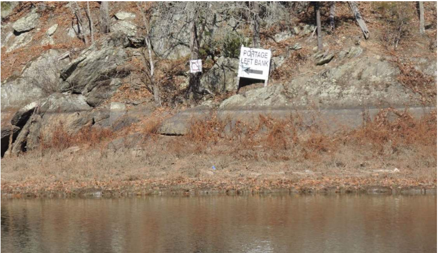
Photo 7-11: Directional sign to portage across the river from the road and portages
