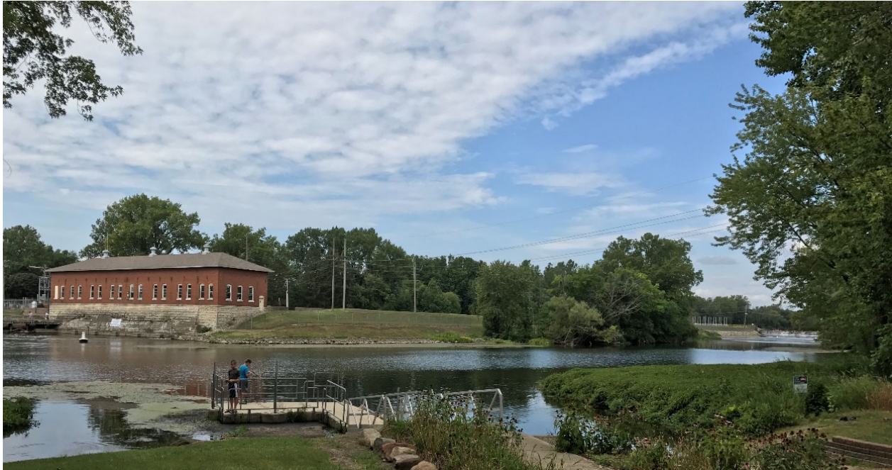
Photo E.10-1 View of Powerhouse from Riverview Park on East Side of River
