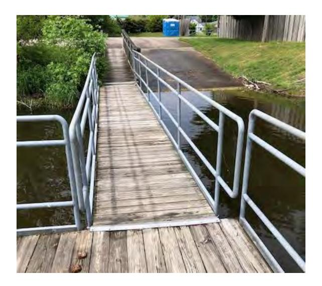
Boat Launch: Wood and metal are in good shape. Restroom in the background is in fair shape. Parking lot is in very good shape. May need some trimming of vegetation.
