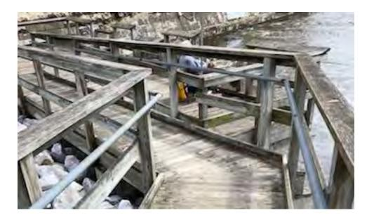
Tailwater Fishing: Wood and metal are in good shape. Needs a trash receptacle (although fisherman pointed out that if they put a receptacle here, people tend to dump their household trash).
