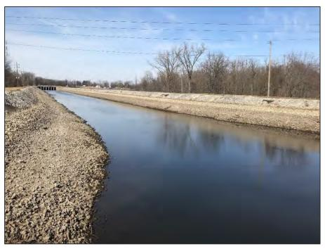
Figure 2. Water level in the head race channel on March 27, 2019. Note stone on channel banks and channel bank toe-of-slope just starting to become exposed. Photo taken at downstream end of head race at power house, facing upstream.
