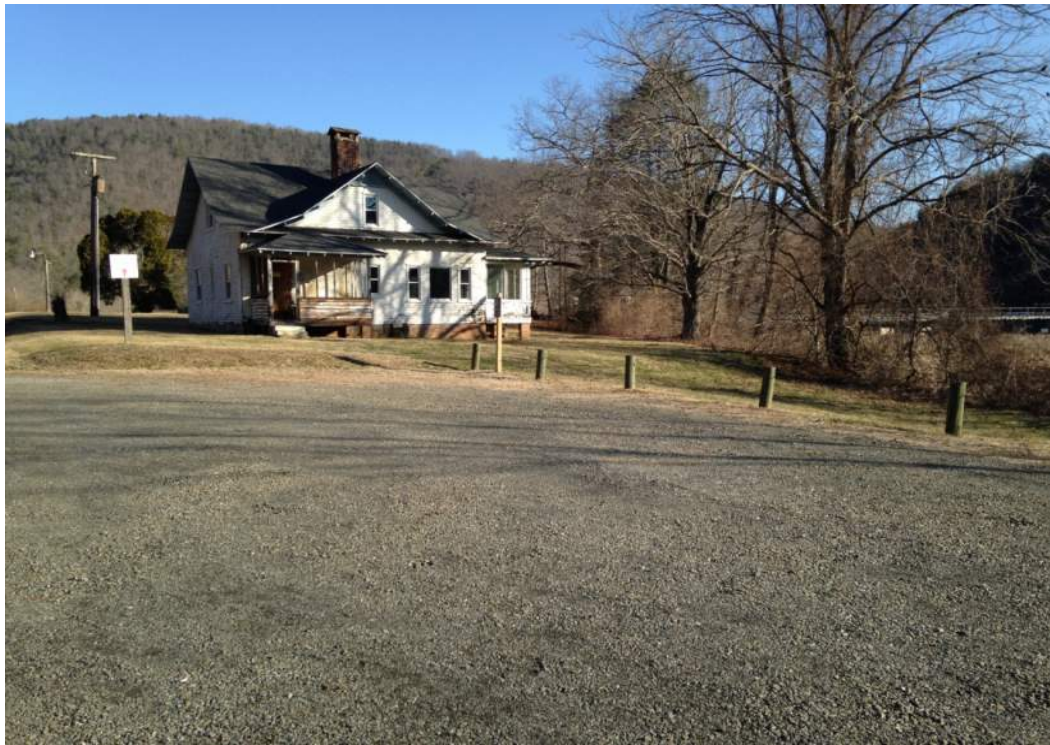
PHOTO 4-7 BYLLESBY CANOE PORTAGE PARKING AREA
