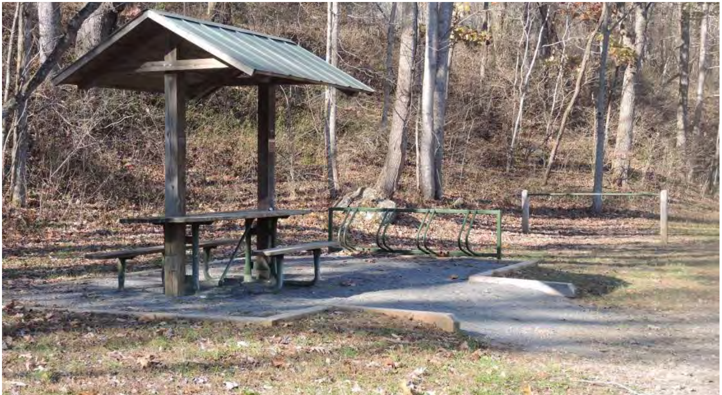
Photo 5-2: Picnic shelter, bike rack and hitching rail
