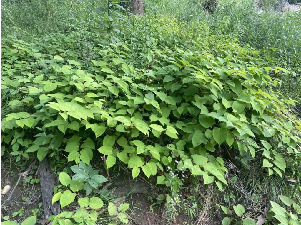
Erosion Area 7; Category “Moderate”
