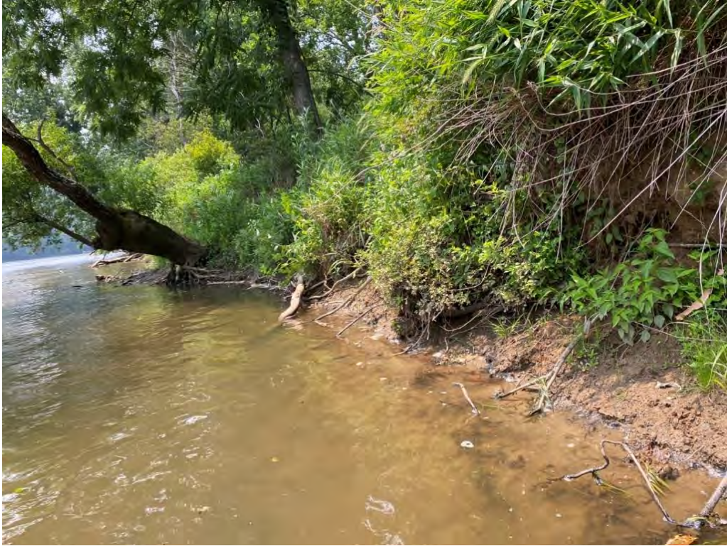
Erosion Area 5; Category “High”
