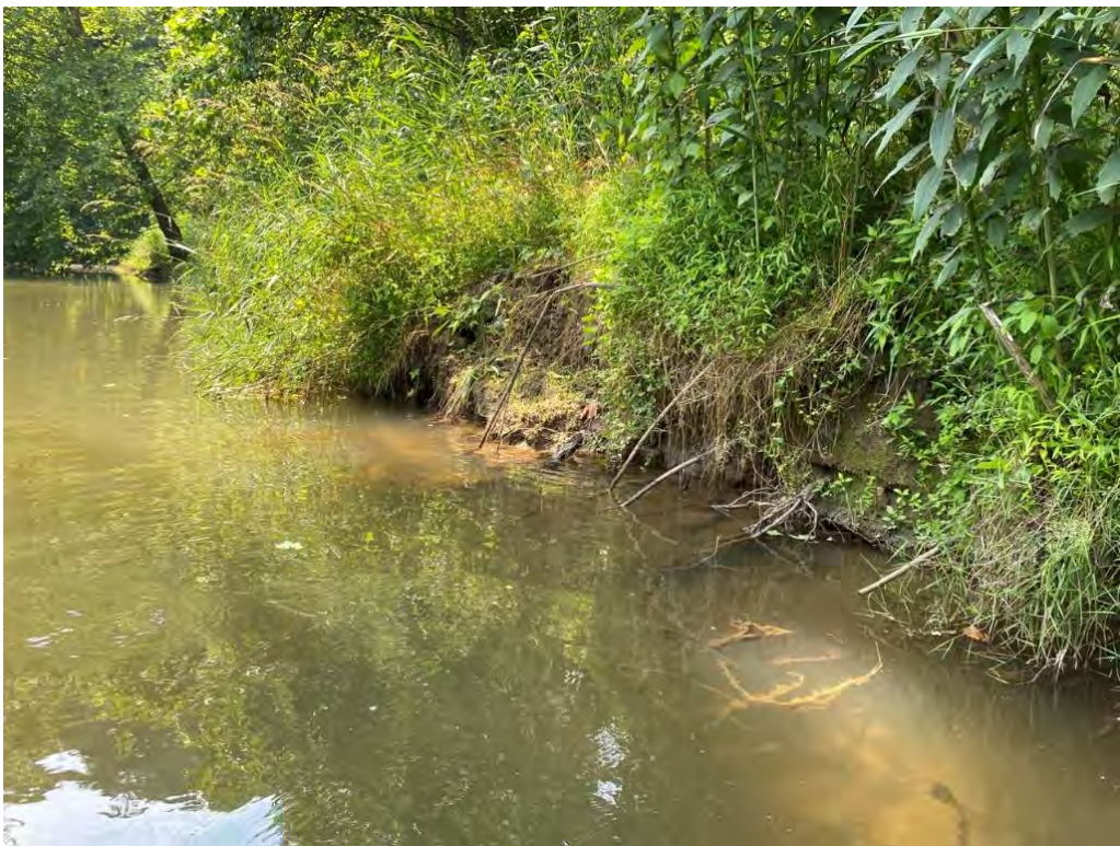
Erosion Area 14; Category “Moderate”
