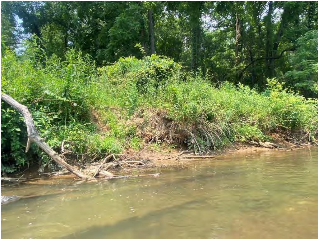
Erosion Area 6; Category “High”
