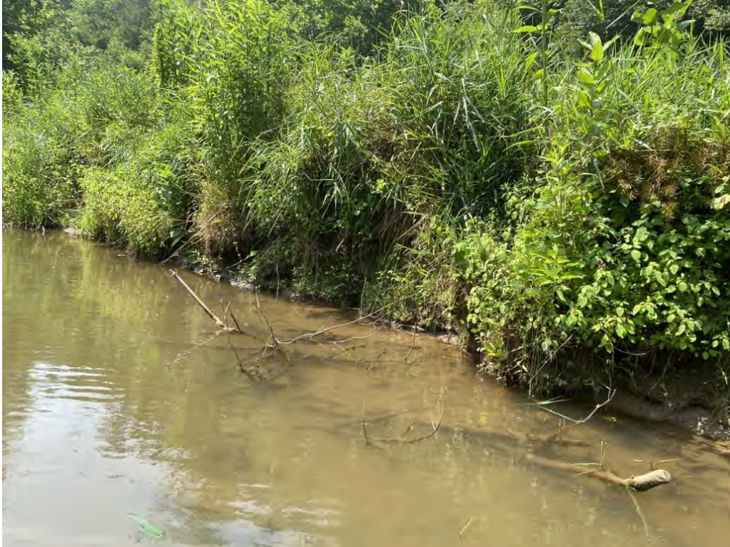
Erosion Area 13; Category “Moderate”
