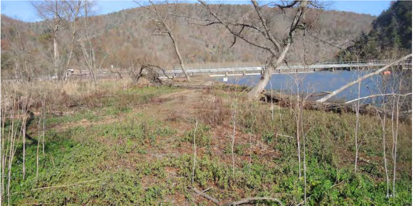
Photo 3-11: Section of trail near the portage take-out is grown over with vegetation and needs to be resurfaced to provide sufficient walking surface and to clarify trail route.
