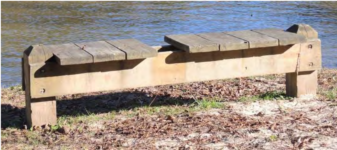
Photo 5-9: Bench with missing slat
