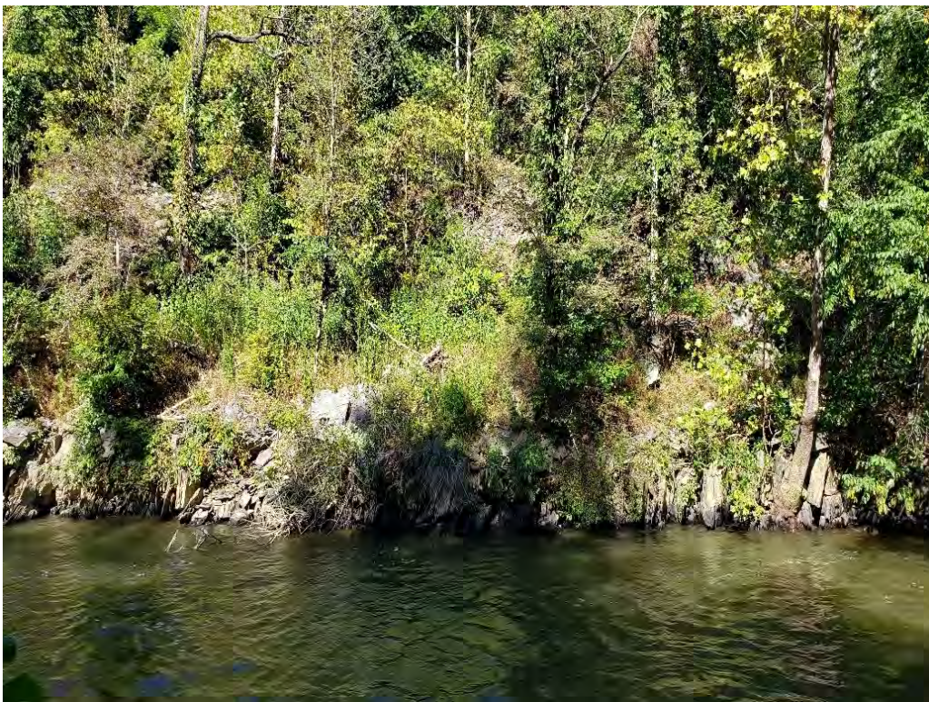
Erosion Area 8; Category “Moderate”
