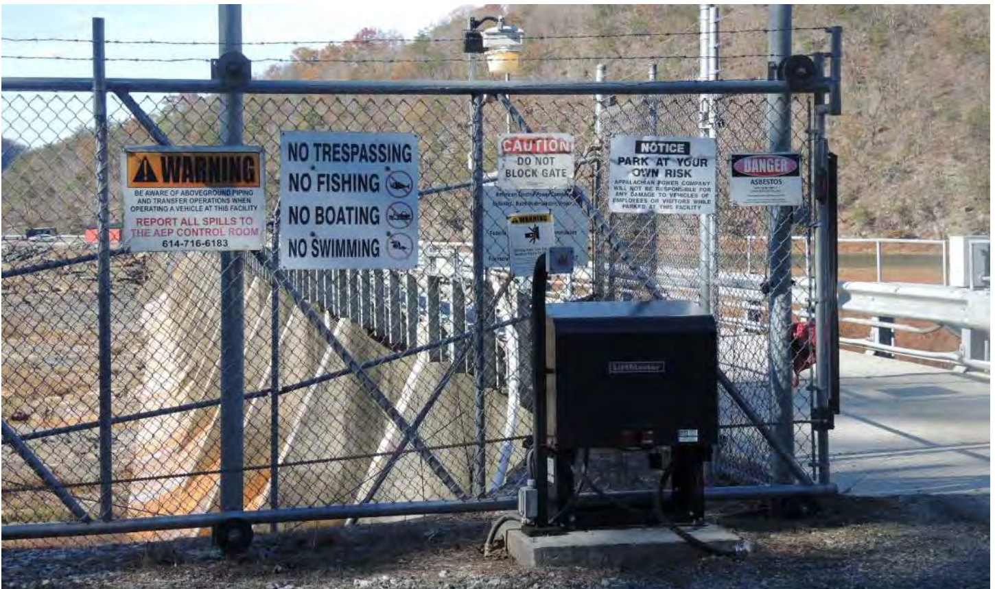
Photo 6-2: Dam gate with regulatory signs
