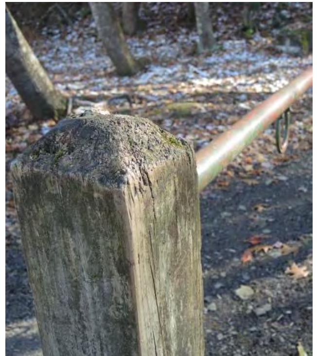
Photo 6-10: Hitching rail with chipped post and faded paint
