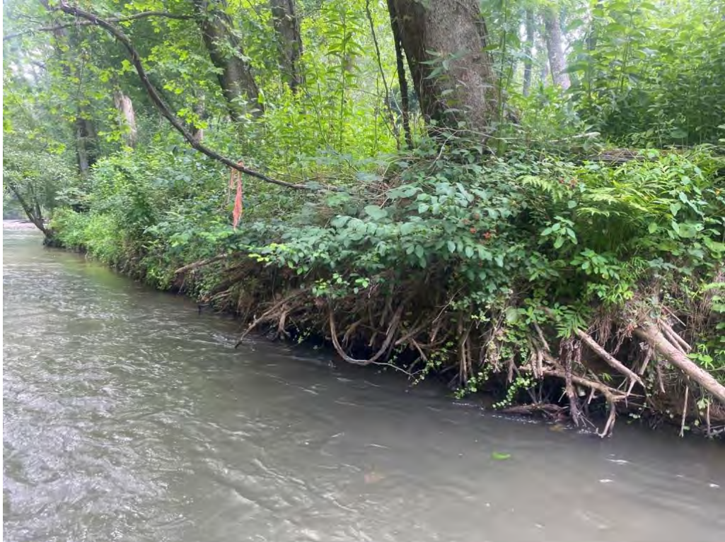
Erosion Area 3; Category “Moderate”
