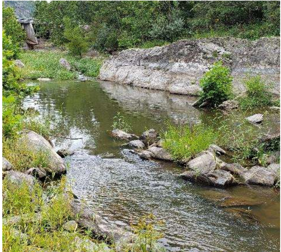
Buck Bypass Reach Side Channel Area 9.9.2020 Leakage Flow
