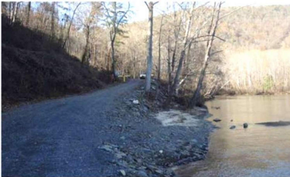
Photo 4-3. Canoe portage put-in and maintenance road accessing it from the parking area
