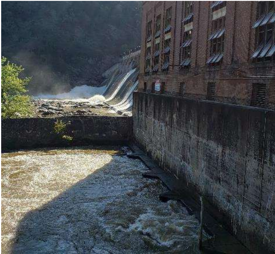
Byllesby Powerhouse and Tailrace (foreground); Main Spillway (background) 8.18.2020
