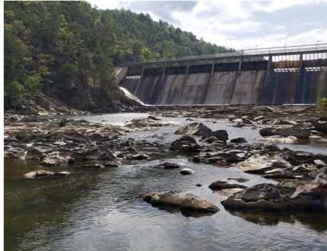
Byllesby Bypass Reach 9.8.2021 Leakage Flow 11 cfs
