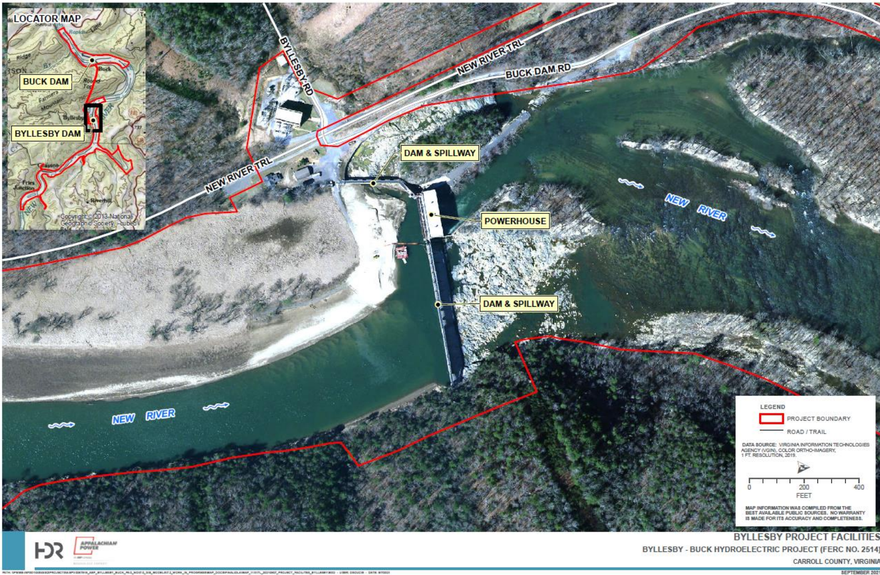
Figure A.2-1. Existing Project Facilities – Byllesby Development
